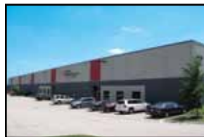
Distribution Center Carol Stream, IL
